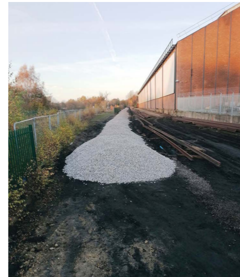
Bottom ballast run out along the headshunt.
