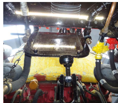
Above right: Newly-installed front buffer beam lighting under test.
