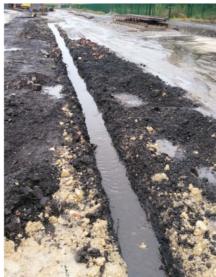
Above: Water flowing freely along the newly formed ditch and on the right more base ballast is run out along the headshunt.
