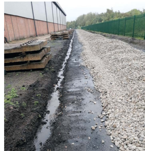
Above: The waybeams being unloaded and right, the heavy rain in October necessitated the provision of a trackside culvert to clear the water from the trackbed.
