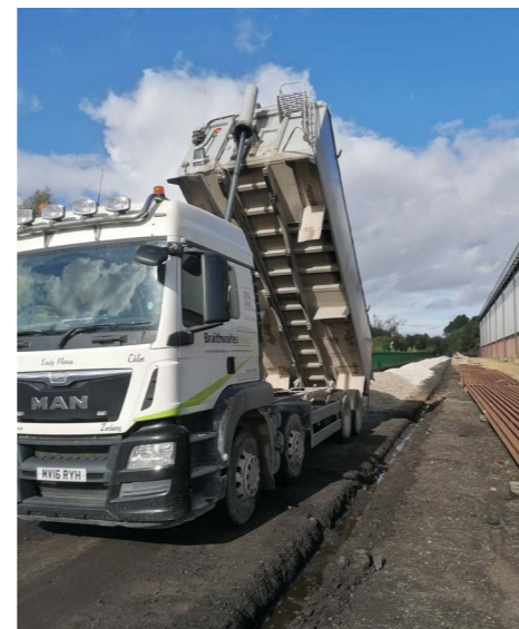
Above: Water flowing freely along the newly formed ditch and on the right more base ballast is run out along the headshunt.
