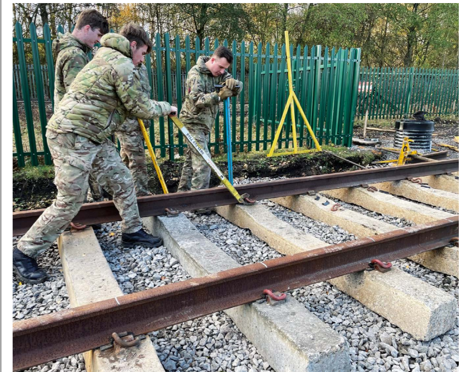
Above and left: Soldiers from 32 Regiment get stuck in laying track and spreading ballast at DLW2.
