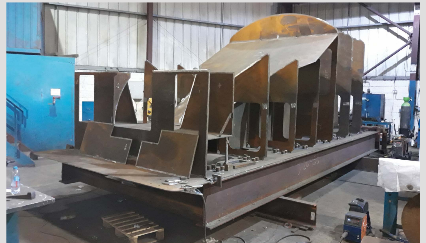
No. 2007's tender taking shape at North View Engineering Solutions.
