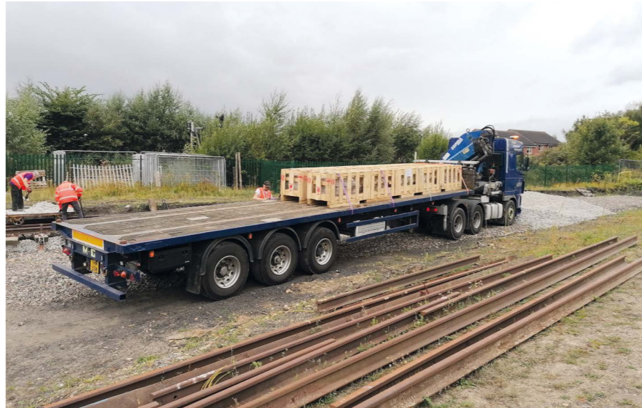
The new waybeams are delivered to DLW2.
