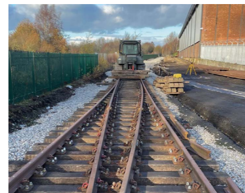
Above and left: Soldiers from 32 Regiment get stuck in laying track and spreading ballast at DLW2.
